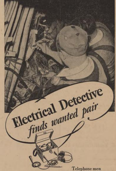
know this piece of apparatus as the 108-A Amplifier. It is an "exploring amplifier," developed by Bell System engineers to identify pairs of wires in telephone cables—some of which contain as many as 4242 wires.
